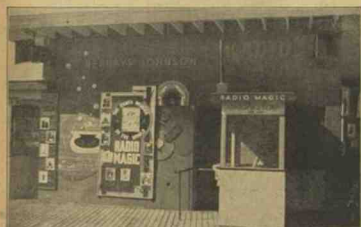
THE THEATER OF RADIO MAGIC at the New York World's Fair utilizes a modern sound system with loudspeakers outside the building and others indoors to provide various sound effects and other features of the performance. The system employed is one of the portable type which operates either from the light lines or a car battery. It will be used when this show later goes on the road a trailer.
