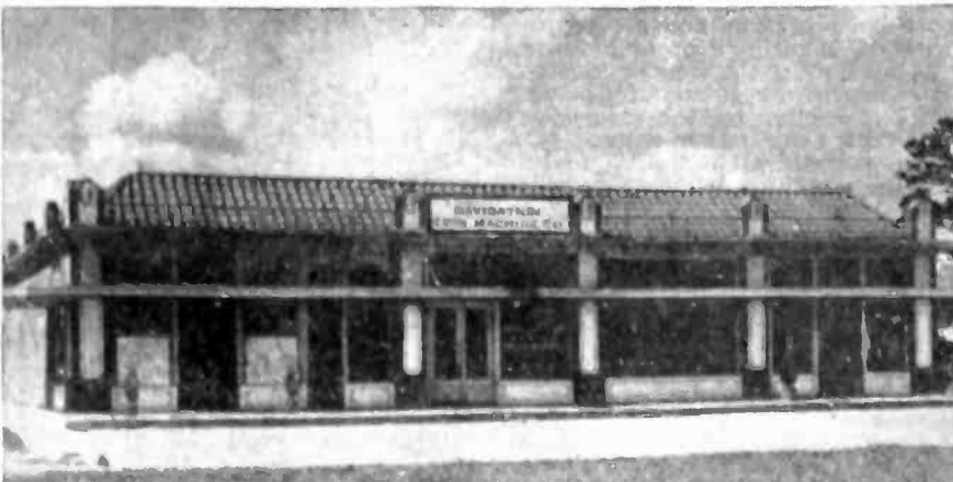
QUARTERS OF NAVIGATION COIN MACHINE CO., Houston, of which M. R. James is general manager. The Navigation firm, James reports, is going along full blast and on several occasions recently it has been necessary to press into service the sidewalk space as an emergency shipping floor.
