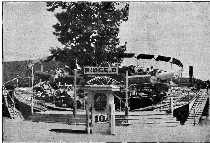
THIS NEW 1938 MODEL RIDE-O RIDE, owned by Orville Walton, has been in operation at Harvey's Lake, Pa. The Spillman Engineering Corporation has gone modernistic in this machine, as will be noted from the lighting panels with indirect lighting and the permanent inclosure panels around the ride, which are considered especially appropriate for park use.
