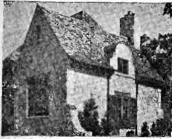
1 This is the House that Jack built.
