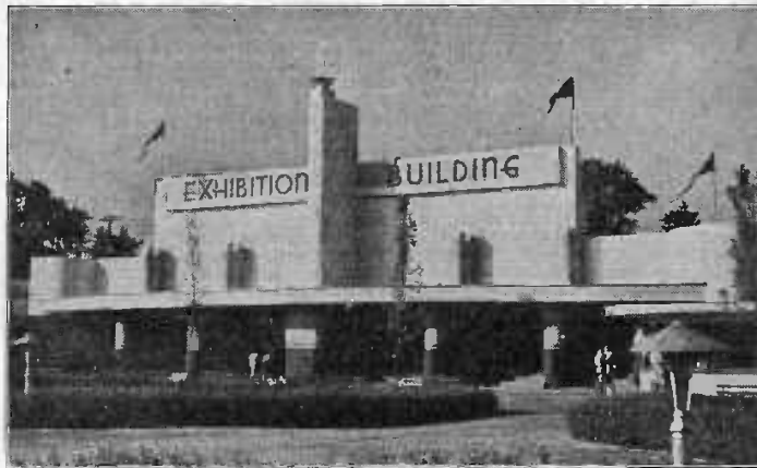
PERMANENT EXHIBITION BUILDING, erected on the Mall in Coney Island, Cincinnati, as part of the reconstruction program following the disastrous January Ohio River flood, is for housing industrial and mercantile exhibits and a start has been made this season. Continuous displays are planned thruout summer and admission is free to park patrons. The modernistic front, with ornate pilasters and novel lighting effects, has curved wings at either end. Interior has more than 40 spacious colorfully decorated booths with striking light combinations. Photo by Myron Benson, Cincinnati.
