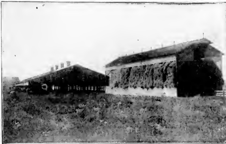
Newly constructed hay barn in which three hundred tons of bright timothy is stored. In the rear is shown the new wagon shed.
