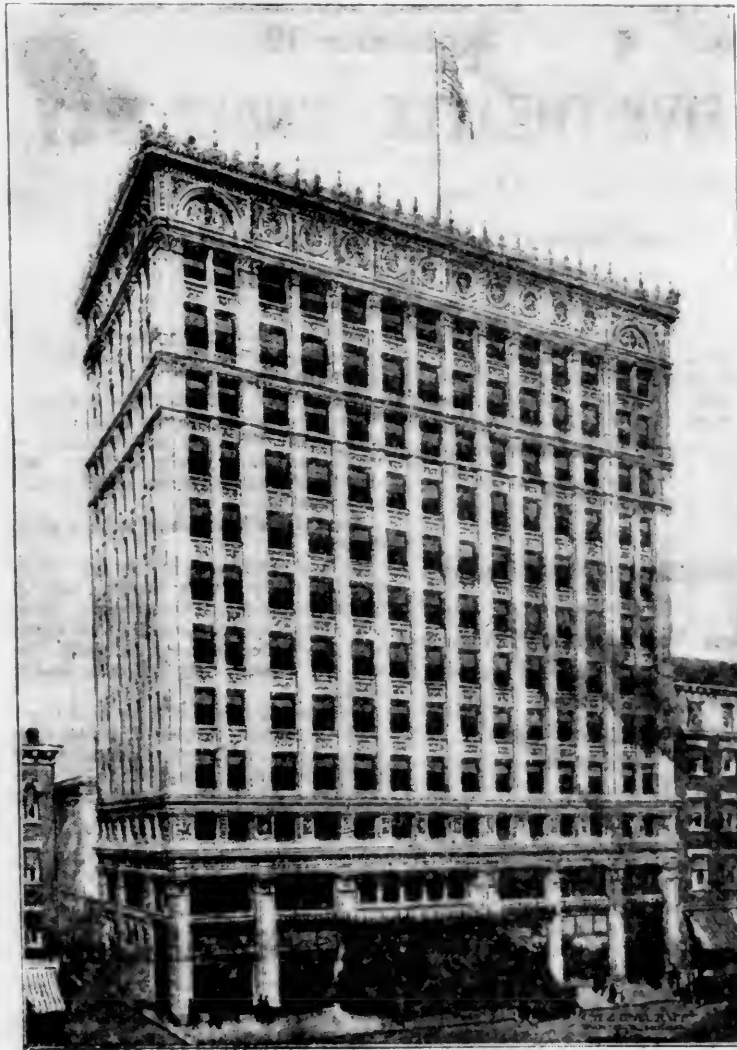
Just completed, at a cost of $1,000,000, this twelve-story structure takes front rank with the largest downtown office buildings in the Queen City. The United Theaters Company, Cincinnati, is owner. The building has a 124-foot frontage on Walnut street, and is 69 feet deep. The exterior is of polished granite and white granite finished terra cotta. The corridor flooring is of art marble and the walls of white marble. Entrance to the offices is the same as the lobby of the theater, around which the improvement has been built. Provision has been made for an enlargement of the playhouse's capacity from 2,200 to 3,600 seats. Ben L. Heldensfeld supervised work on the improvement and is serving in a similar capacity for the two new Shubert houses in Cincinnati, soon to open.
