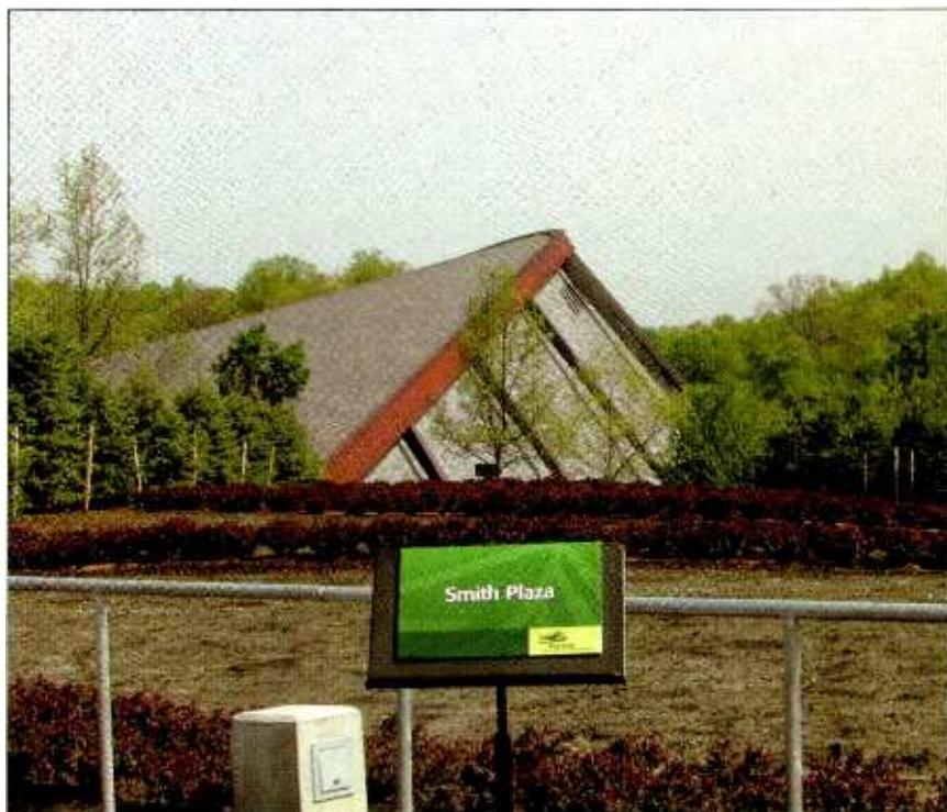
In Bloom. Renovations, including 1,106 additional reserved seats and 3,624 lawn spots, are complete at the Blossom Music Center. There are plans for further development of the grounds surrounding the venue.
