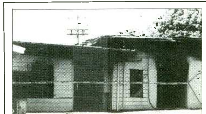
KMXI's studios were taped off following the fire.
