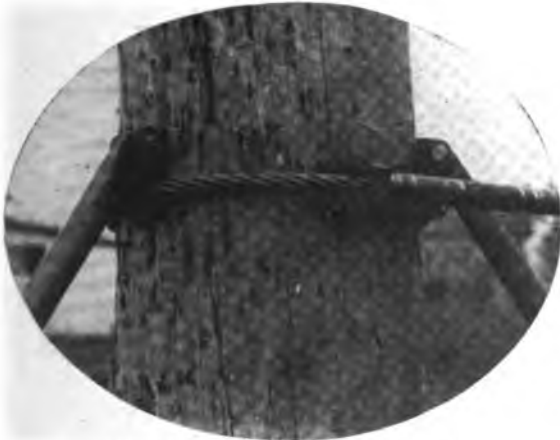
VIEW NO. 1—SHOWING CABLE GRIP.
