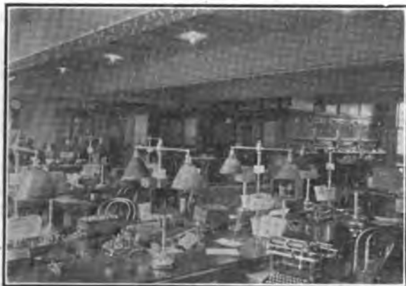
VIEW OF THE OPERATING ROOM.
