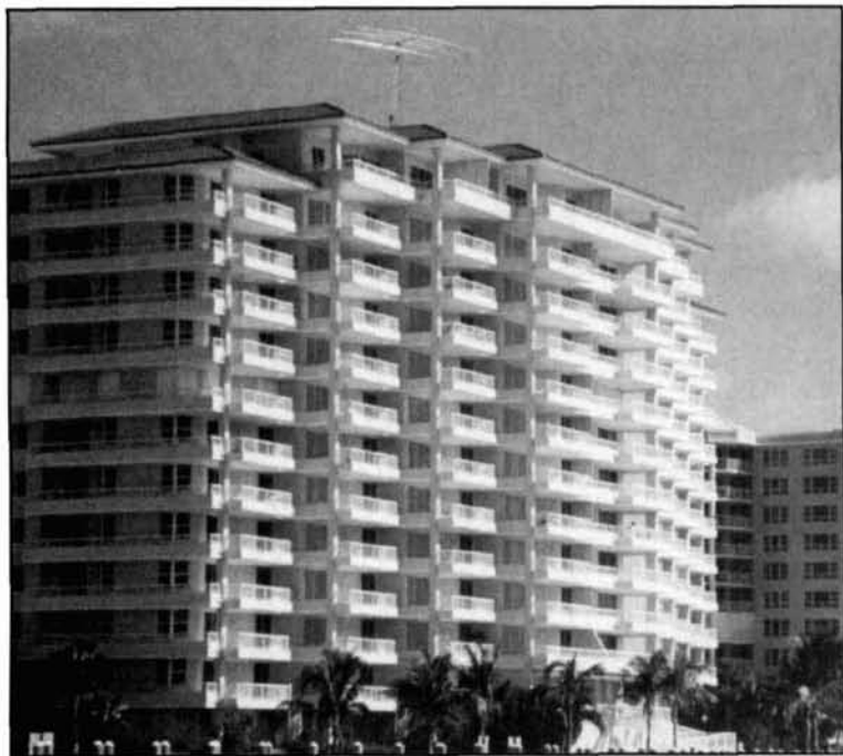
Photo B. Eight-element, log-periodic antenna atop the Cap Marco Merida Condominium, Marco Island, Florida (160 feet or 50 meters above ground level). It is connect to ham station KA2WEU/4 located in the penthouse below.
