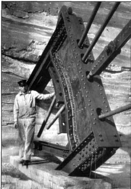
Photo F. Massive early Guy Anchor ("dead man"). This one is anchoring four guys. "Twenties vintage. Source: Dr. James E. Brittain.
