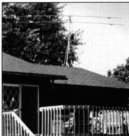
Photo C. A low-profile tripod installation..
