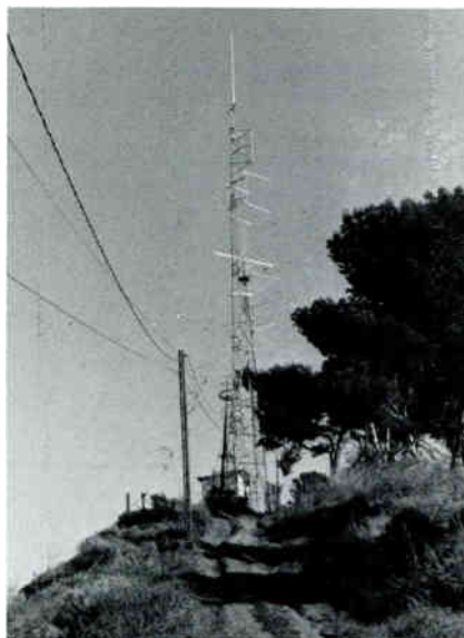
Tower at the head end sight in the Ventura foothills of California
