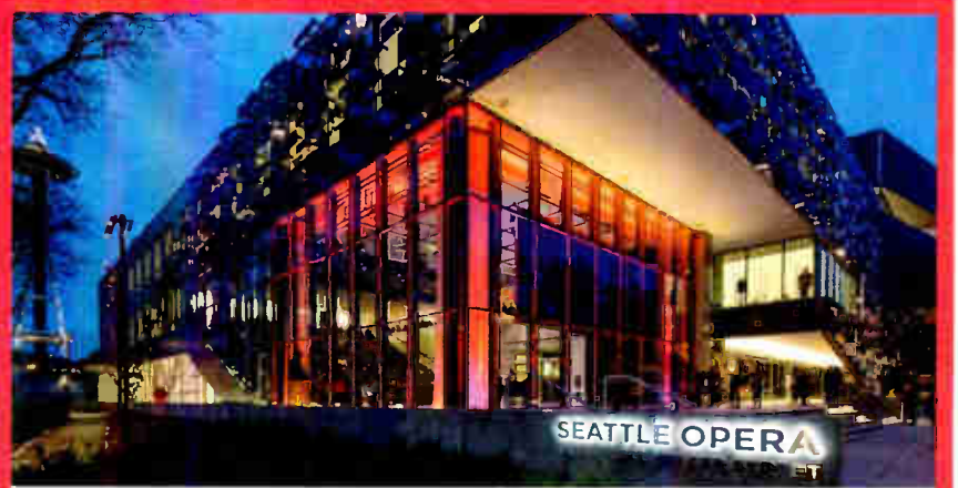
The studios of iconic classical music outlet KING-FM are within this new Seattle Opera building near the Space Needle (far left).
