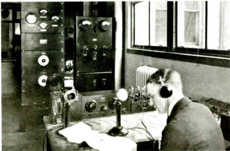
Operator Fred Lathrop is at the controls of WWJ in 1922. The Western Electric 1-A 500-watt transmitter is rear left, with its electrical control panel at right. The desk contains only a microphone, audio amplifier, radio receiver and a wavemeter (frequency monitor). A room behind the transmitter contains a motor-generator set and banks of storage batteries, which supply DC power to the transmitter; power rectifier tubes had not been invented.
