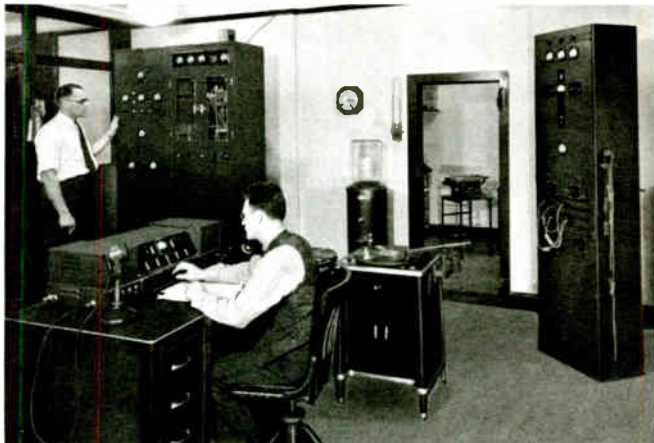
WWJ's ultra-shortwave "Apex" station W8XWJ broadcast from 1936 to 1940 on 41,000 kHz. Chief Engineer C.H. Messer attends to the 500-watt high-fidelity AM transmitter in the Penobscot Building. Carroll Leedy operates the control console. W8XWJ later became W45D, one of the nation's first FM stations (now WXYT-FM).
