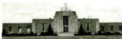
In 1936 WWJ raised power to 5,000 watts and moved from the News building to this new transmitter building and tower on Eight Mile Road. Like the studio building opened that same year, the transmitter building was designed by Albert Kahn. Its granite block façade was highlighted by leaded glass windows towering above the doors.
