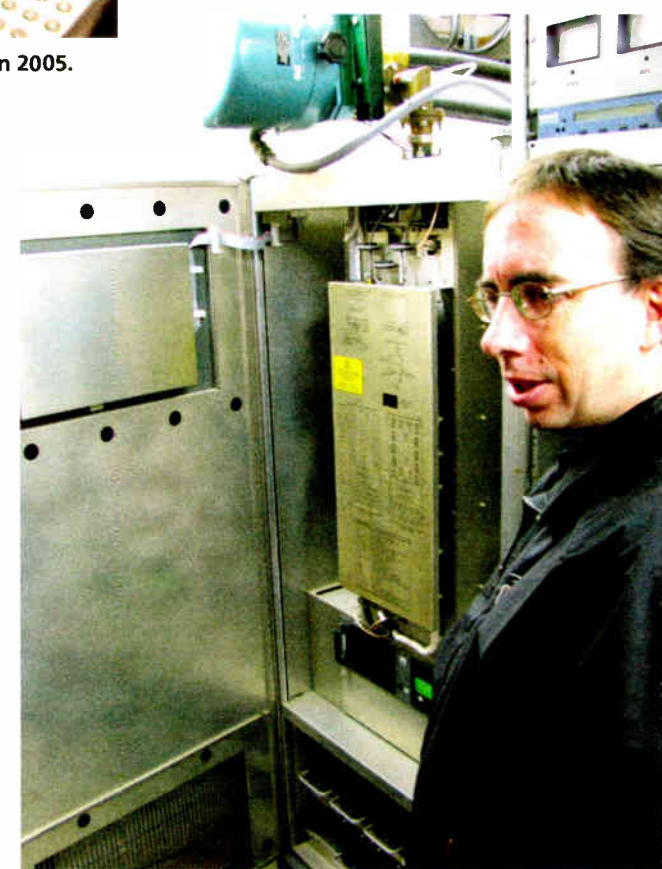
Welton inspects a newly installed V5 in Wisconsin in 2010.
