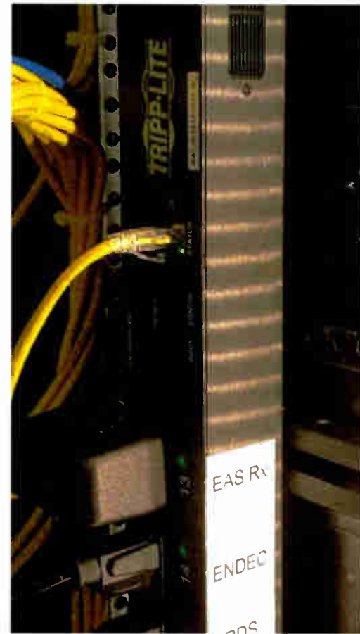
Fig. 3: Tripp-Lite has added a network connection to its power strips for monitoring and control.
