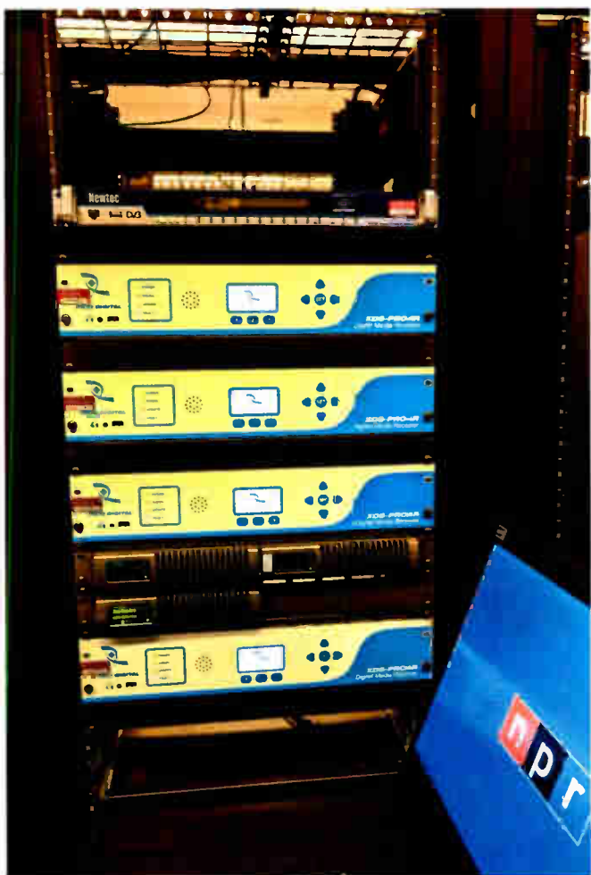
Fig. 2: Satellite DVB2 modulation and four ATX Pro4R receivers for testing. The rack also includes a rack-mounted KVM for system setup.
