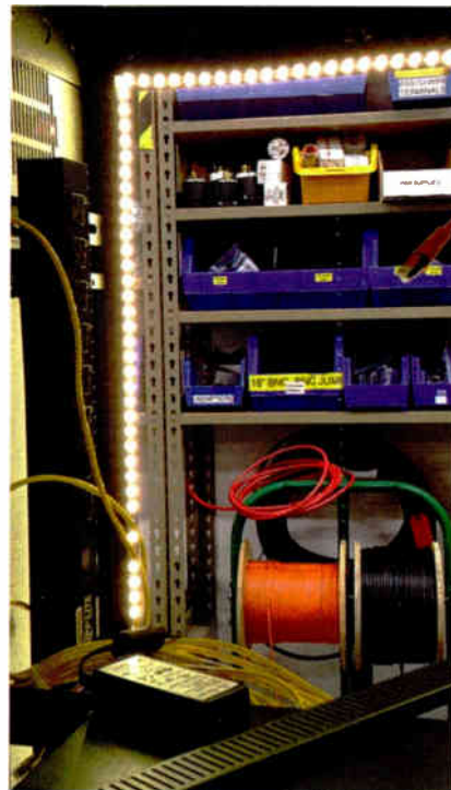
Fig. 3: The LEDs efficiently light an equipment rack.
