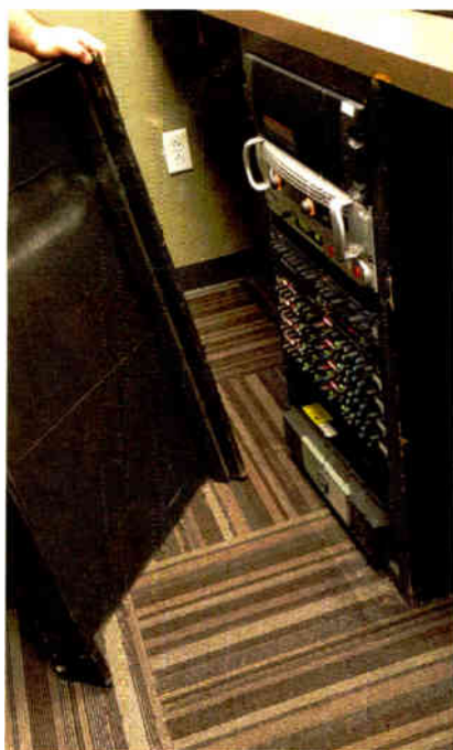
Fig. 1: The cover snaps in place to keep curious fingers from sensitive control knobs.
