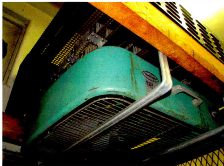
Fig. 1: Here, our perspective is turned up to look at the ceiling, where the fan has been mounted to blow upwards.
