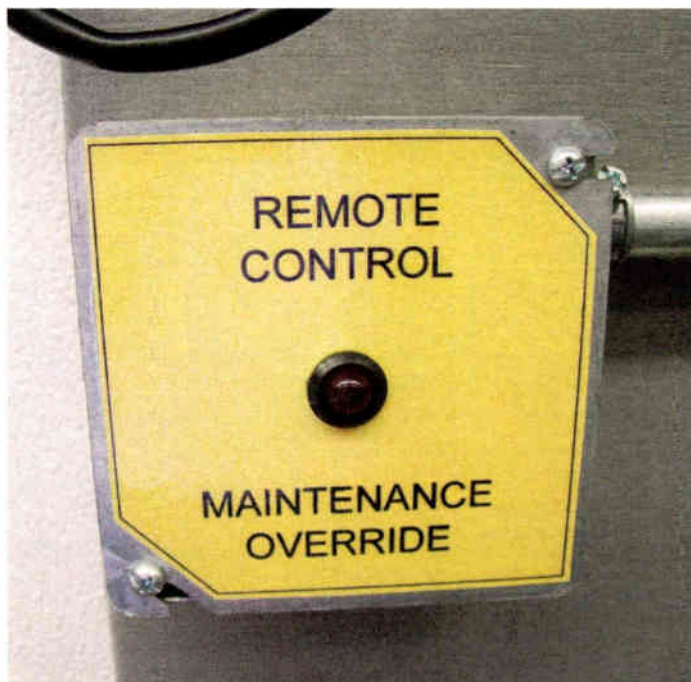
Fig. 4: Place this warning box by your door as a reminder to reset the remote control.
