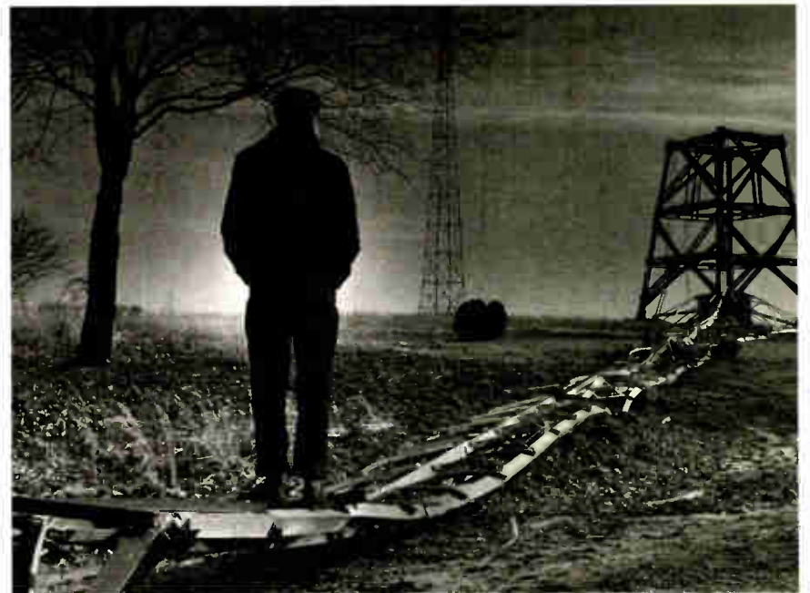
WAWZ has faced its share of weather-related troubles over the years. Rea Crawford is shown in 1950 inspecting damage from a hurricane that toppled the upper portion of one of the station's self-supporting towers. WAWZ was an AM at that time.
