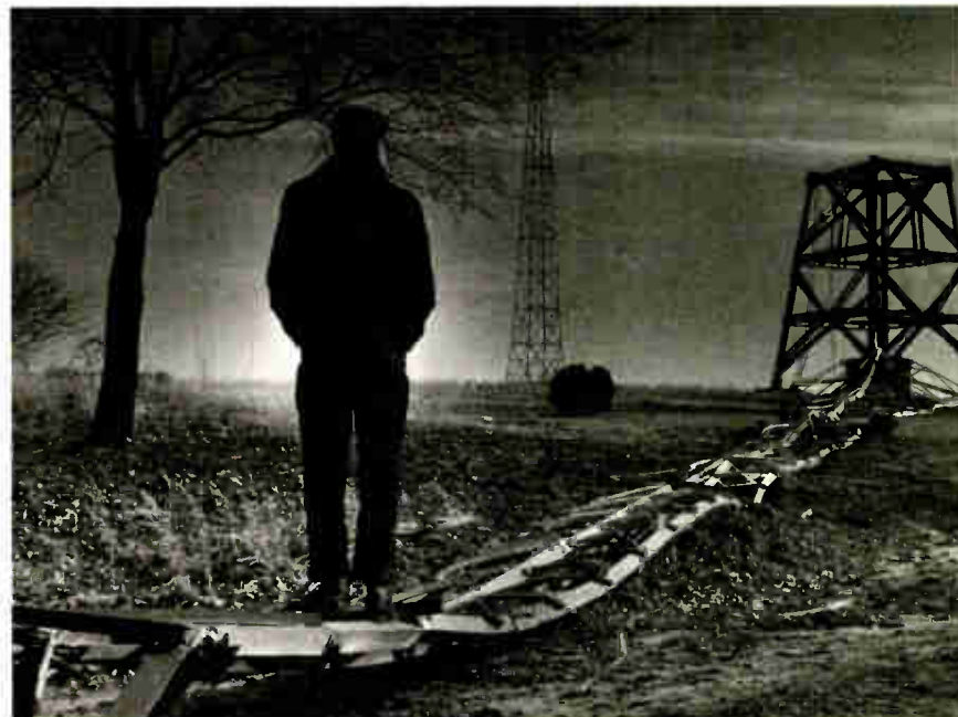
WAWZ has faced its share of weather-related troubles over the years. Rea Crawford is shown in 1950 inspecting damage from a hurricane that toppled the upper portion of one of the station's self-supporting towers. WAWZ was an AM at that time.
