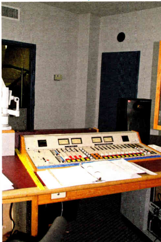
Hubbard Radio's WTOP(AM/FM) is the Local Primary station in the nation's capital. It has a complete off-site backup studio and reciprocal agreements with other stations to share studio space if needed. Its three transmitter sites provide redundancy; the main back-up facility is shown.
