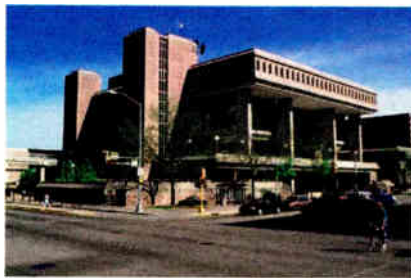
An urban office building in Madison, Wis.
