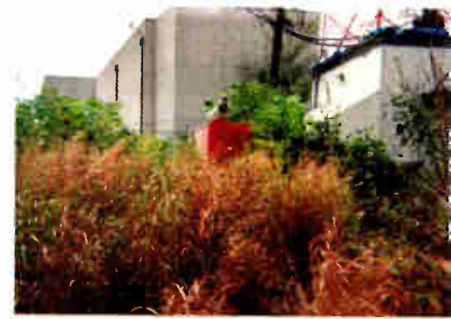
Fig. 2: Overgrown weeds and bushes are a fire hazard. They also can serve as cover for a thief or vandal.
