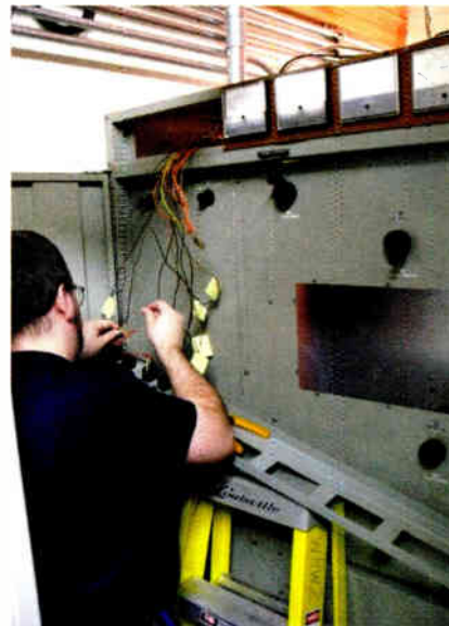
The author works on rebuilding the front control panel of the Gates FM-10H3.
