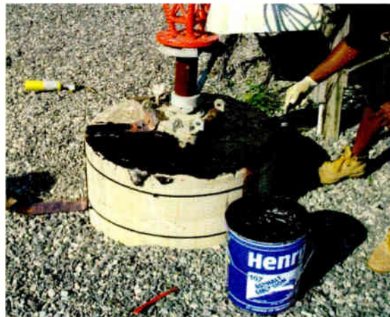
Fig. 2: The tar can be applied easily using a trowel.
