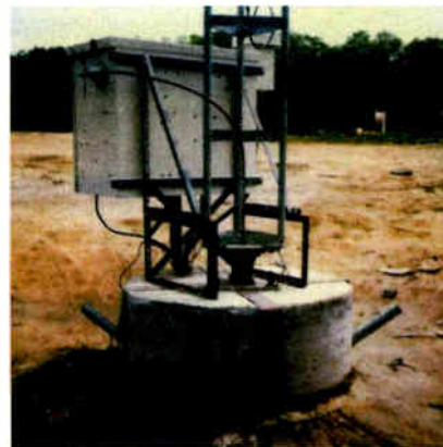
Fig. 3: Jerry Arnold points out that the steel framework supporting the ATU is bolted to the concrete tower base directly. If the ATU is struck by lightning, the surge could explode the concrete base.
