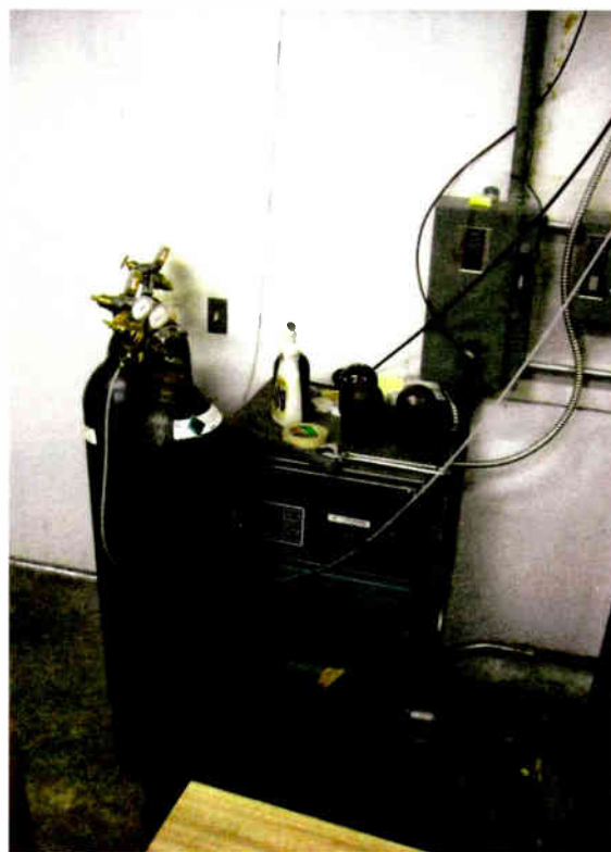
Fig. 1: Test your knowledge. How well does this site conform to good engineering practices?
