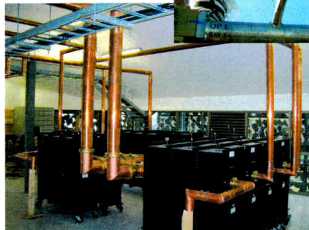
The room was designed for the Dielectric manifold combiner system, shown.
