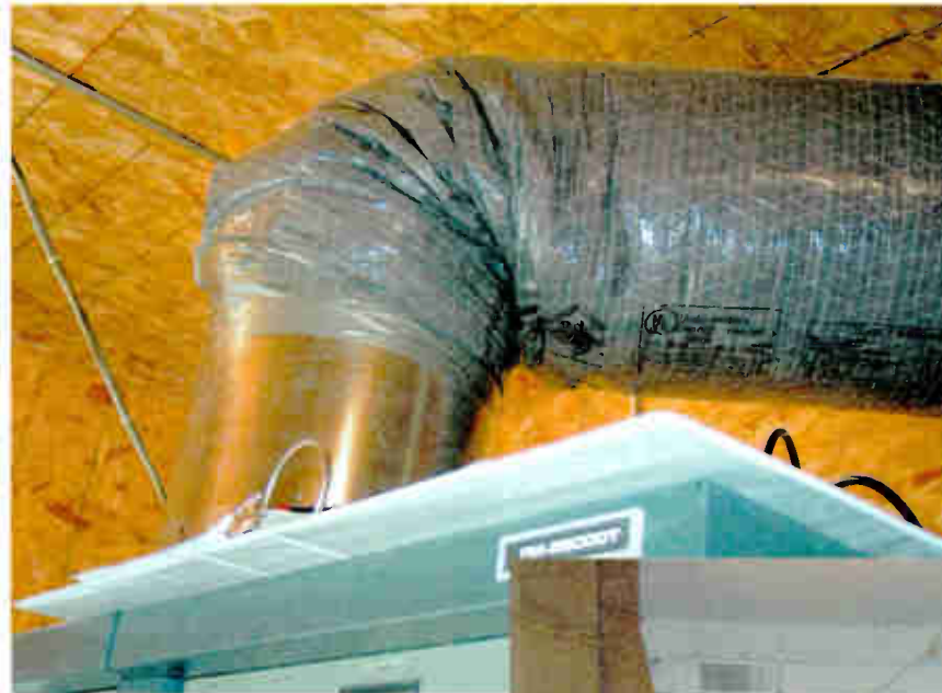
Fig. 1: Avoid constrictive ducting on transmitter outputs.
