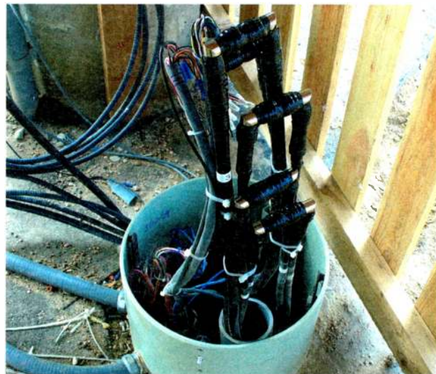
Completed cable splices in the telco pedestal.
