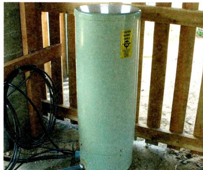
The 14-inch-diameter pedestal provides a secure, dry and accessible environment for the splices.
