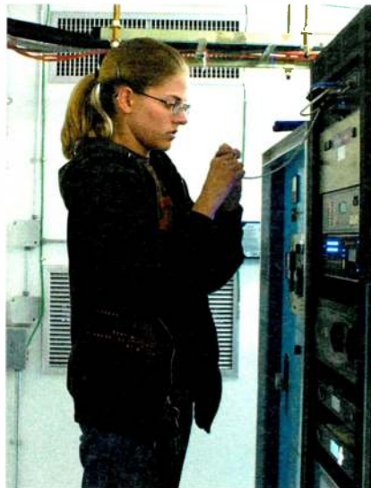
Amanda Alexander wires up the Ethernet switch.
