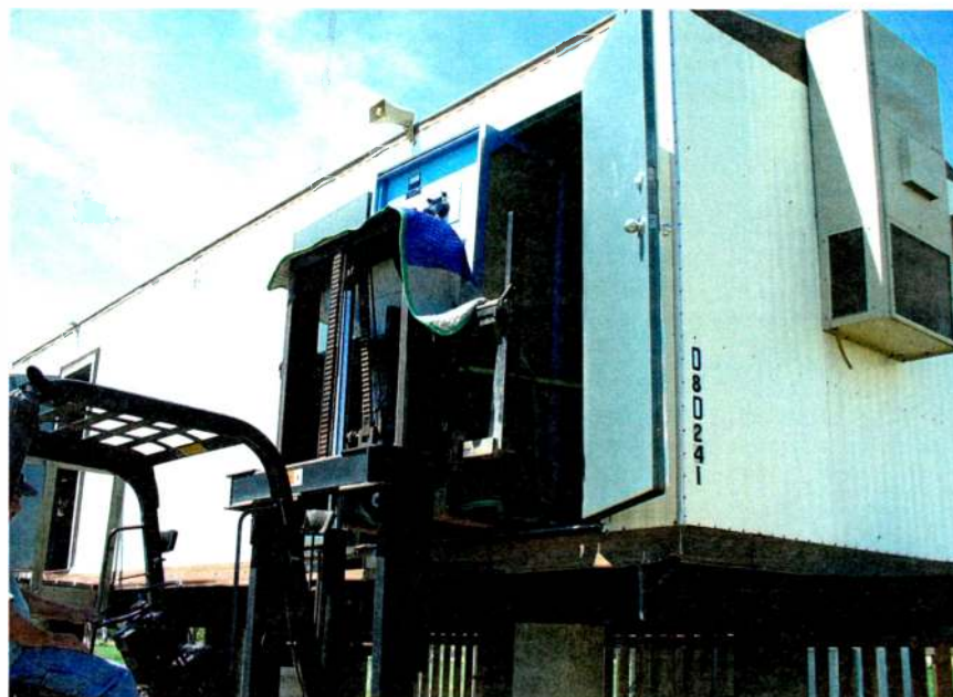
The phasor is removed from the old building by forklift.
