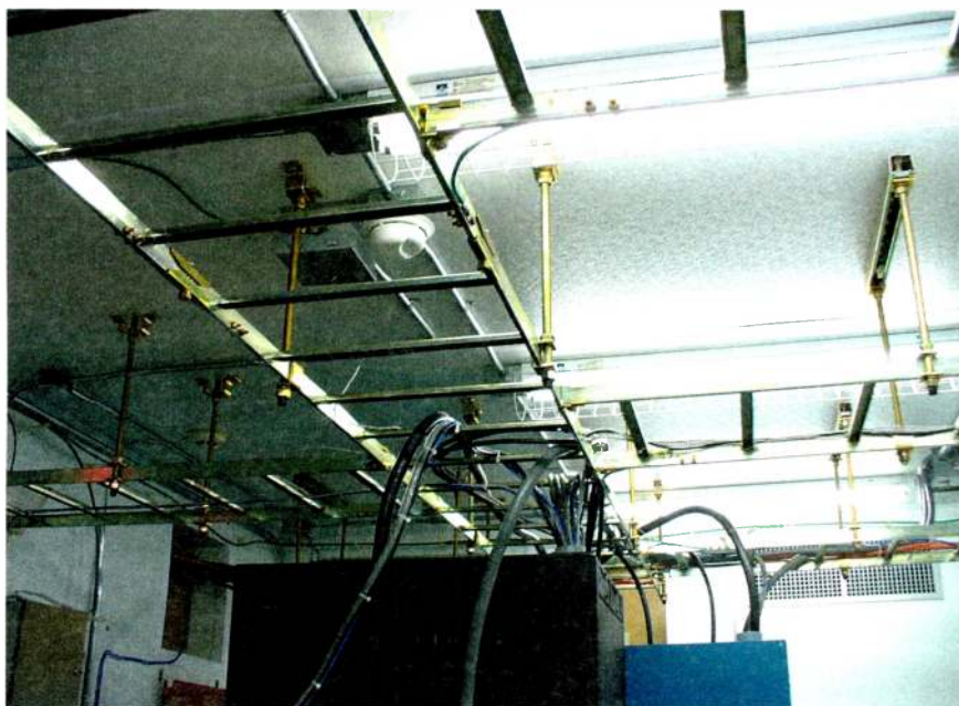
The supplied overhead cable ladder made cable routing and management a snap.
