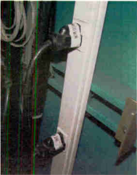
Fig. 3: Don't pull the wrong plug. Label it!
