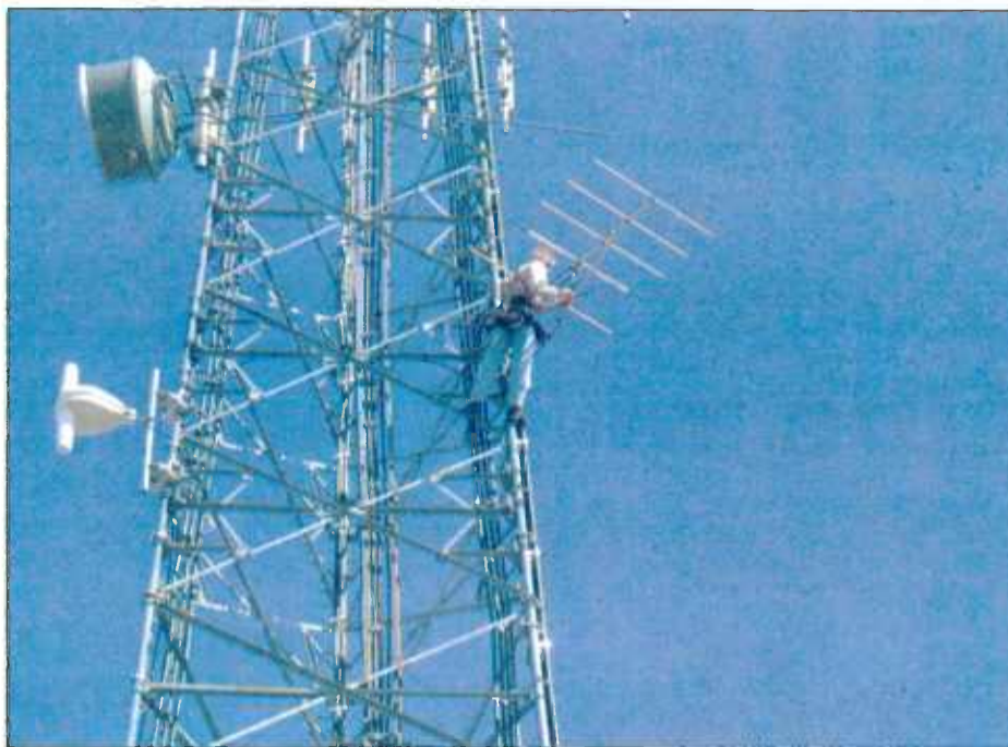
Clarke Boynton of Cardinal RF Systems aligns the North Adams receive Yagi.
