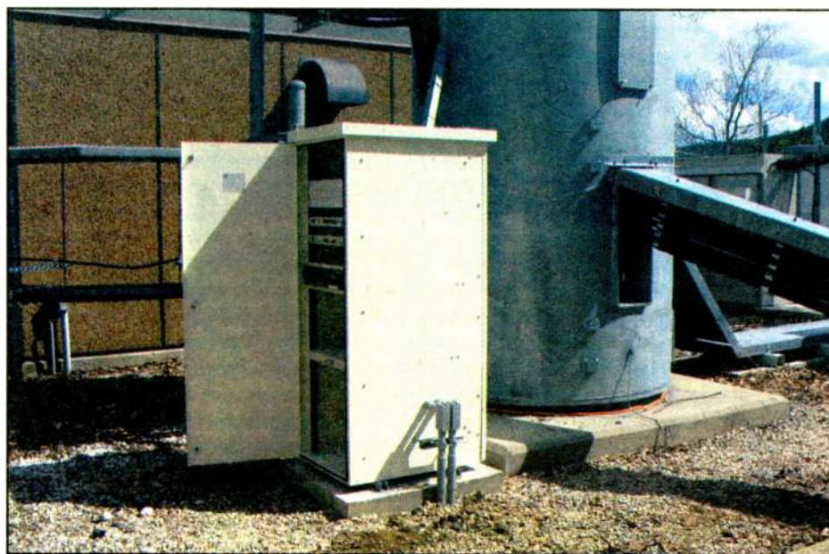
A simple, clean translator consisting of a BE exciter in a Kintronics cabinet.
