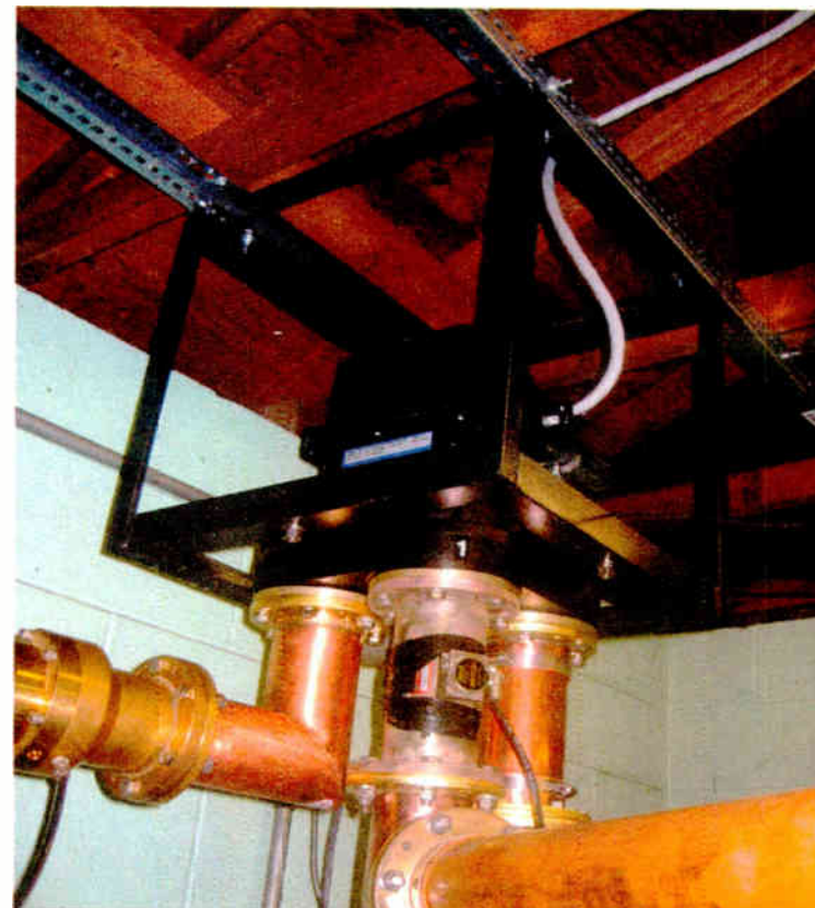
Fig. 3: Switches can be mounted vertically with this bracket.
