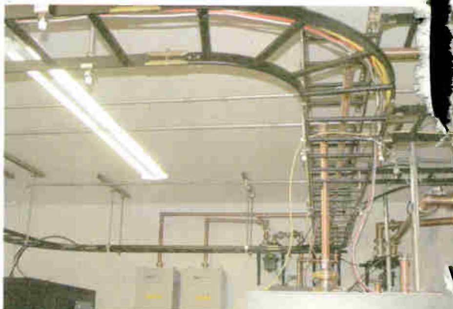
Fig. 2: Level electrical and RF plumbing for a neat installation.
