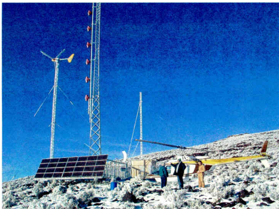
A combination of wind and solar energy powers KRNG's 8,000-ft transmitter site in Wadsworth, Nev.
