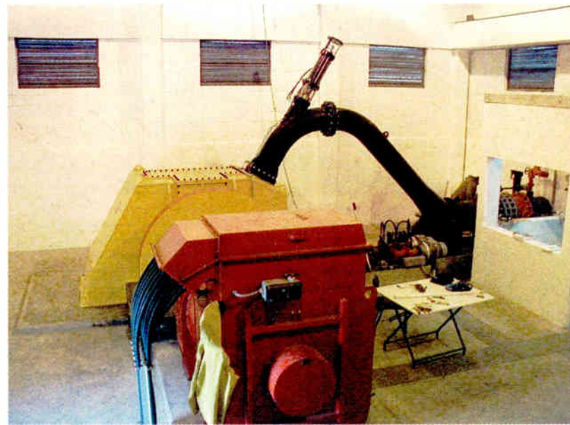
The turbine and generator of HCJB's 2 MW Loreto hydro plant, completed in 2002.
