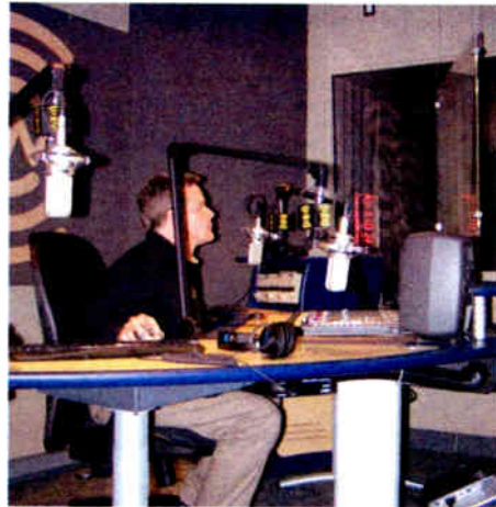
Zandar FusionPro MultiViewers are used by XM for digital signage and display of images including live video, audio and computer signals. One is hanging at right
