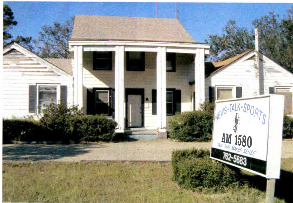
WPMP's building was one of the few structures in Pascagoula that didn't suffer a watery storm surge. Winds took their toll, however. This photo shows the station with its new roof.
