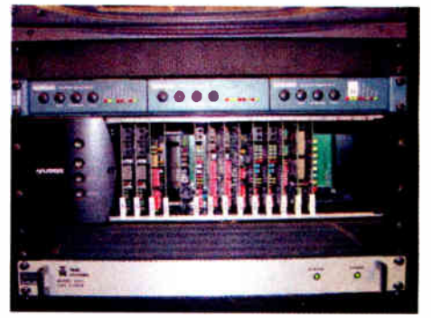
Simmons Media Group in Salt Lake City is using Harris Intraplex SynchroCast digital multiplexers to interconnect three stations.
