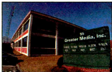
Greater Media installed Axis network cameras and video servers in a security application in Boston.
