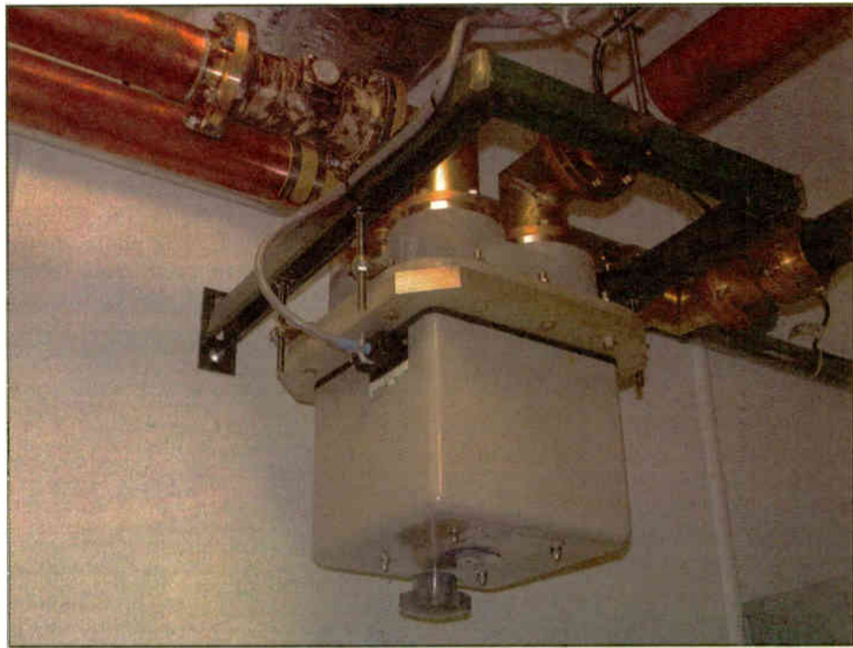
Fig. 3: Anchor the strut with lag bolts to secure the installation.
