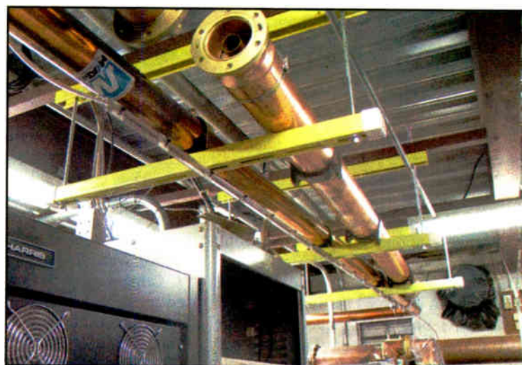
Fig. 4: Painted Kindorf stands out from the gray steel ceiling.
