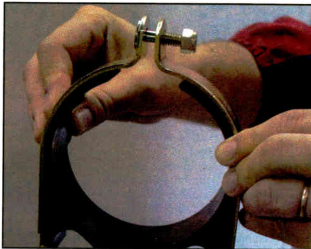
Fig. 3: Mark Bohnett supports his line runs with a rigid conduit system.
