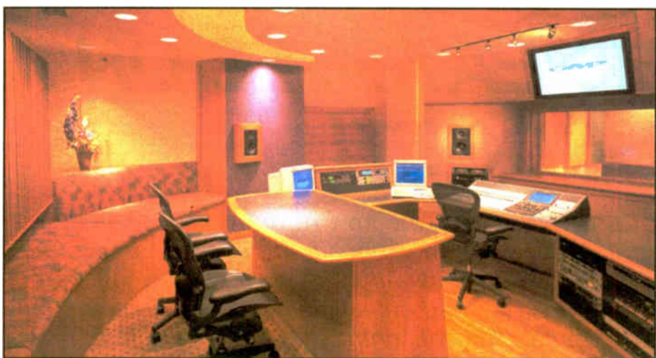
This control room furniture is installed at Gap Digital, a Wheaton, Ill., radio programming production complex designed by Walters-Storyk Design Group. To minimize reflections that may cause comb filtering at the mix position, no furniture installation is above 48 inches.
