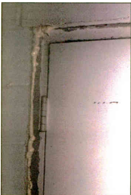
Fig. 1: Seal doorframes with expanding foam to keep nature out.
