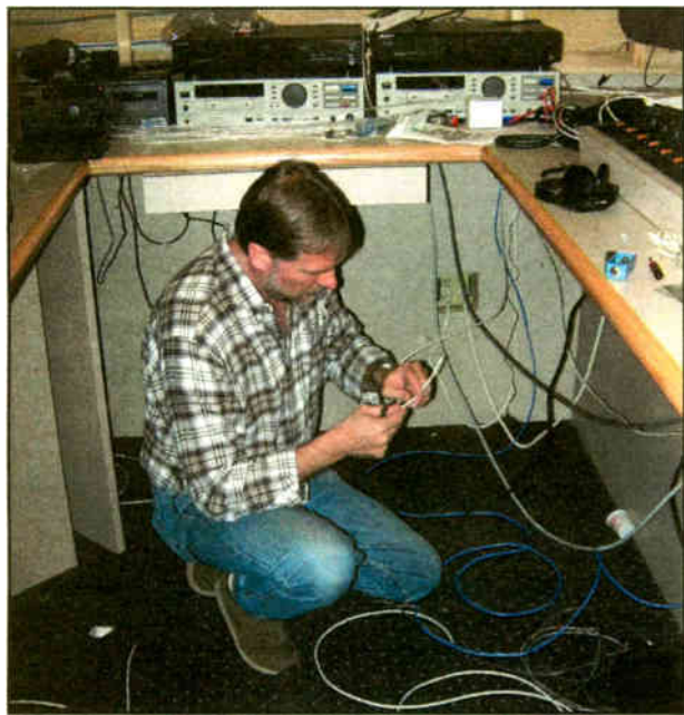
During construction, Assistant Engineer Randy Davis works on studio wiring.
