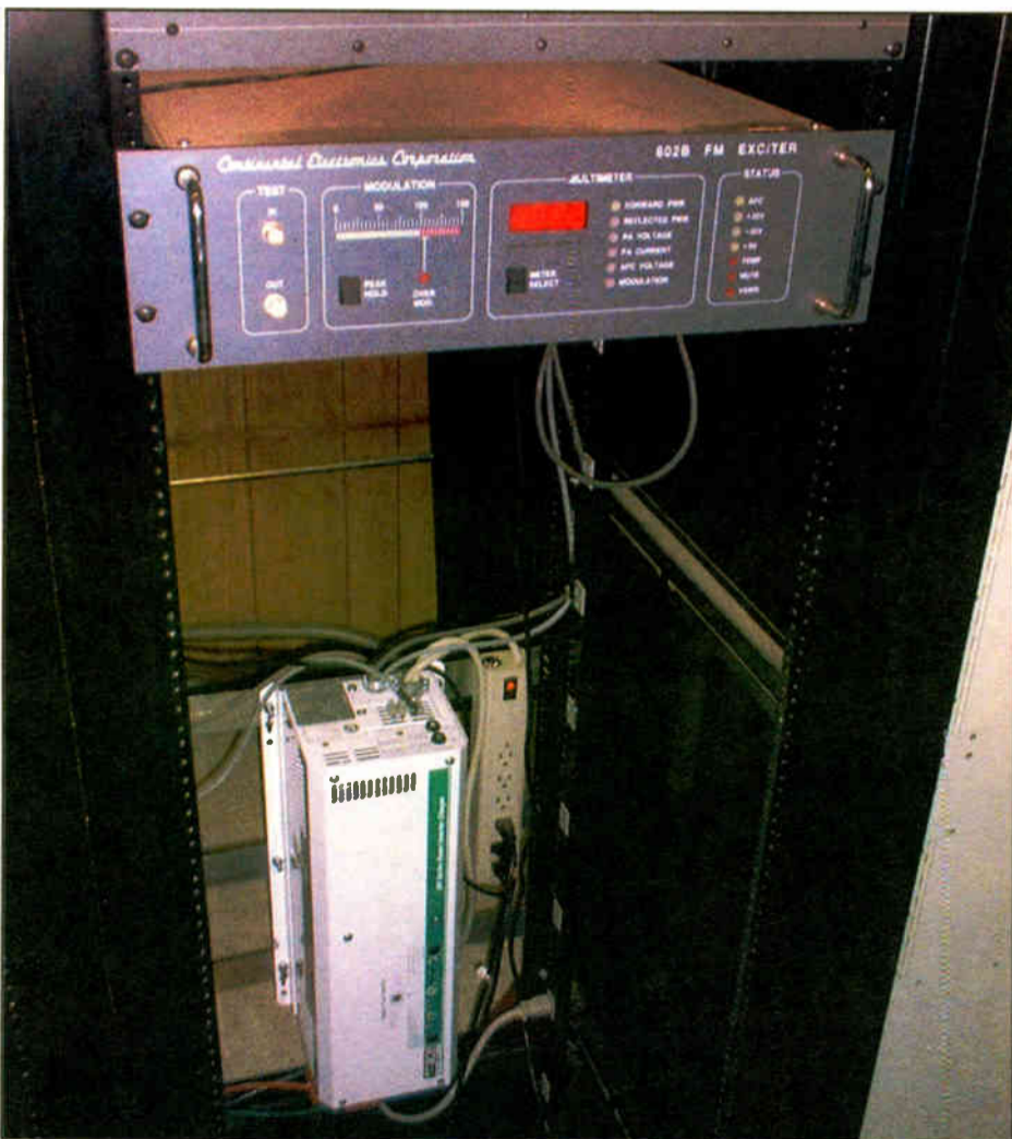
The Model DR1524 Trace unit requires a 24-volt DC input and can provide 1 kilowatt of continuous AC power.
