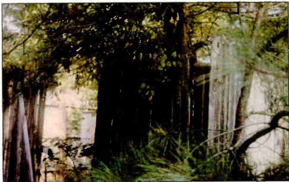
Fig. 1: The pine tree inside this tower fence has pushed right through the wood.
