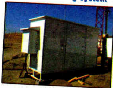
KAFY Radio Bakersfield, Ca 3-Tower 1/5kW DA-2 970KHz
