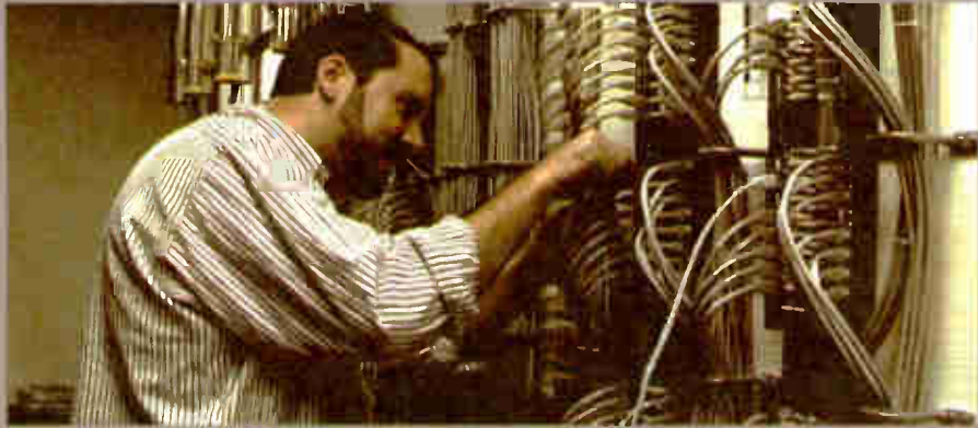
Jeff DePolo wires StudioHub engineering wall in Roanoke, Va.
