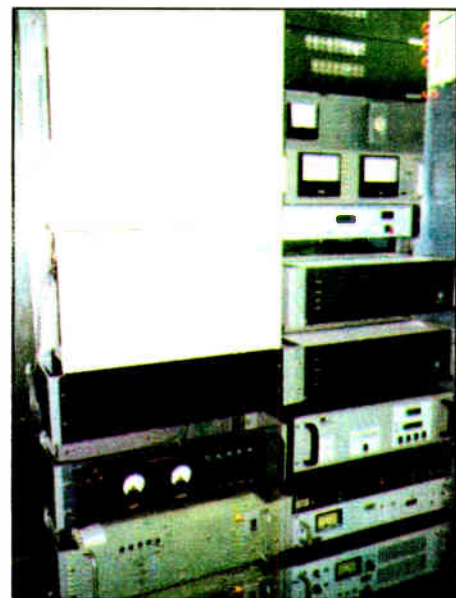
Inside the White Tank Site
