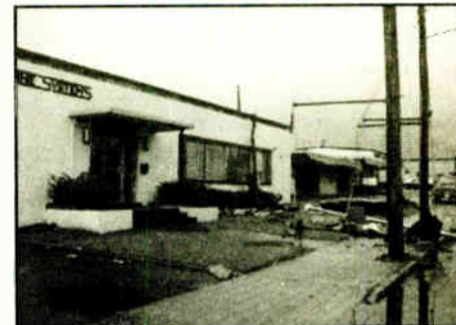
Storm Damage at the Sine Plant
