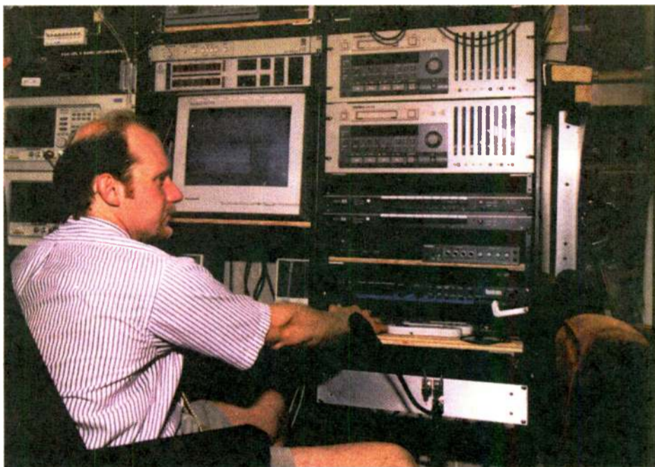
Mission Control: Inside the DAB Test Van
