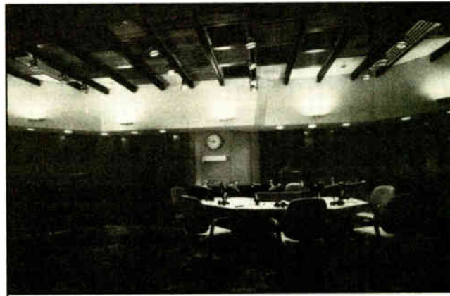
RPG Diffusors are an integral part of WQXR's studio acoustic ceiling treatment.
