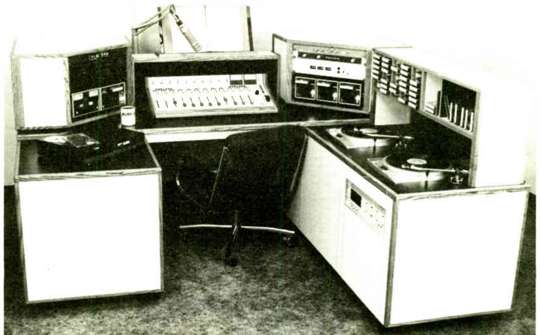
This studio was installed 5 hours after it was delivered.
